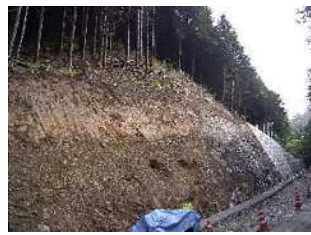
①法面清掃
