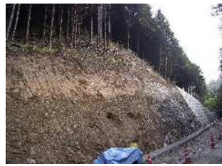
①法面清掃
